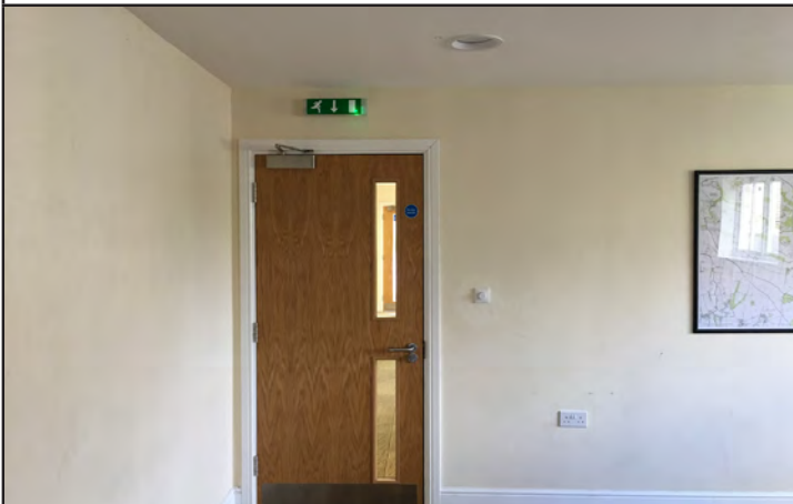
Door above into corridor
