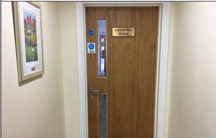
Fire door into Litchfield Room
