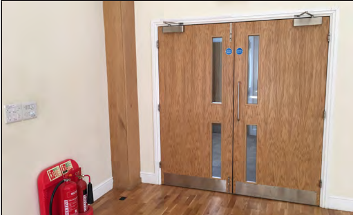
Hall Entrance Double doors into Corridor & Fire Equipment
